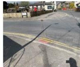
Existing dropped kerb / informal crossing point. May require tactile paving to be provided.
